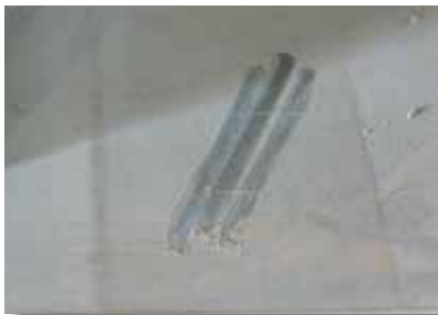
Detail of the dust deposited inside a galvanized sheet metal duct stored in a job site
