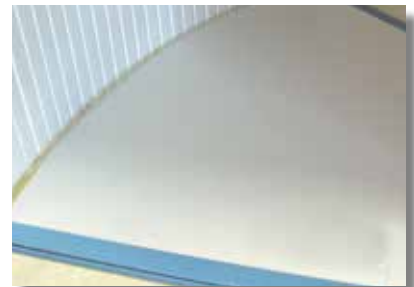
Detail of the dust deposited inside a careplus P3ductal duct stored in a job site
