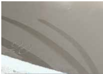
Detail of the dust deposited inside a smooth indoor P3ductal duct stored in a job site
