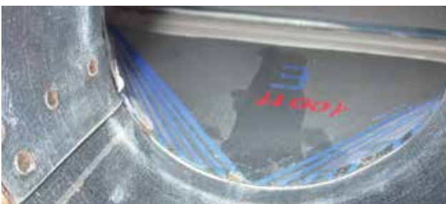
Detail of the dust deposited inside a smooth indoor P3ductal duct stored in a job site
